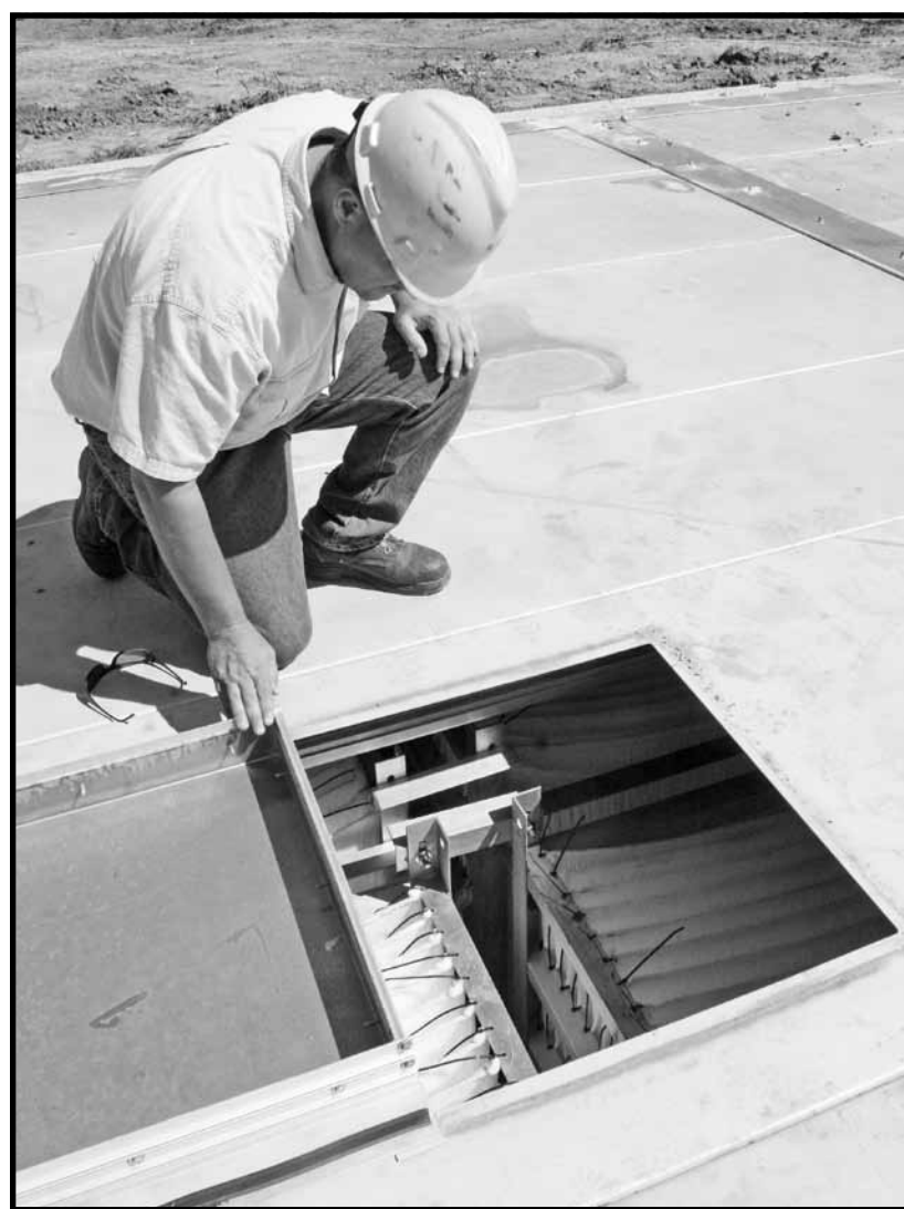
(Photo by Clara Osten) Garry Poutre, Public Works Superintendent, inspects the Media curtains in the new wastewater treatment plant.
